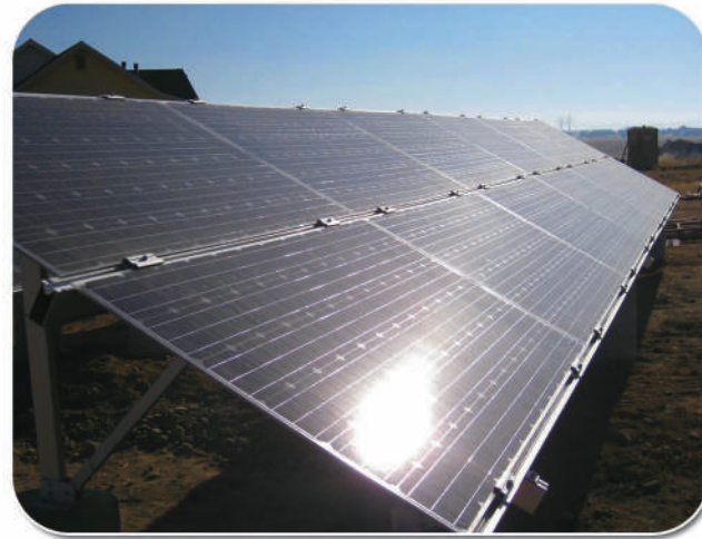
50KW SFS-GM-01B Ground Cement Mount System(USA)
