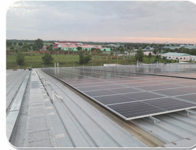
2MW SFS-PR-01 Tin roof solar mount (Vietnam)
