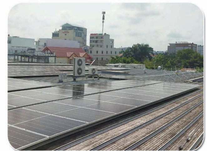
900KW SFS-PR-01 Tin roof solar mount (Vietnam)
