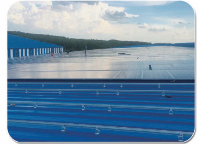
4 MW SFS-PR-01 Tin Roof Clamp Racking (Vietnam)
