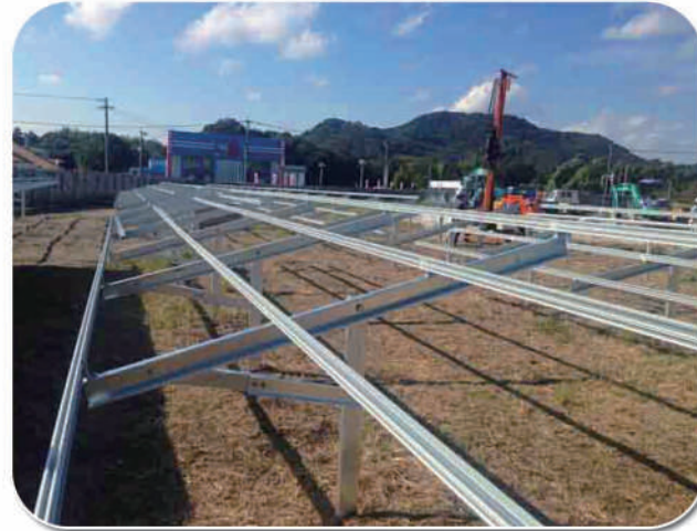
3.5MW SFS-GM-04 Pile Ground Mount Structure(Japan)
