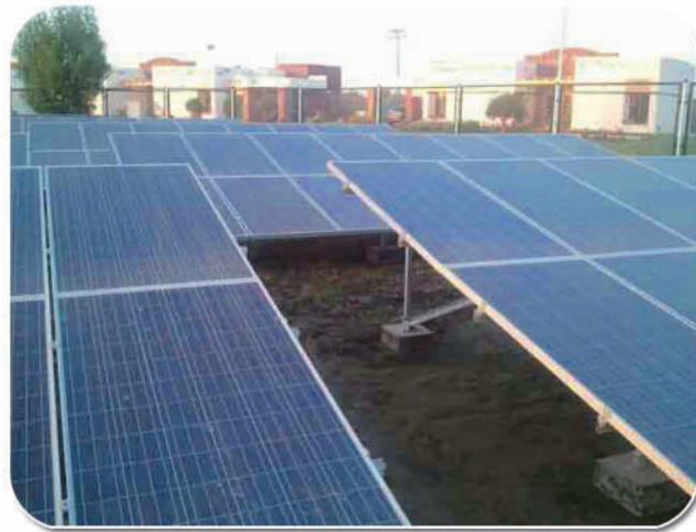
1.4MW SFS-GM-01 Concrete Base Mount System(Kazakhstan)
