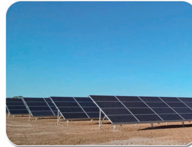
250kw SFS-GM-02B Ground Screw Mount System (Australia)
